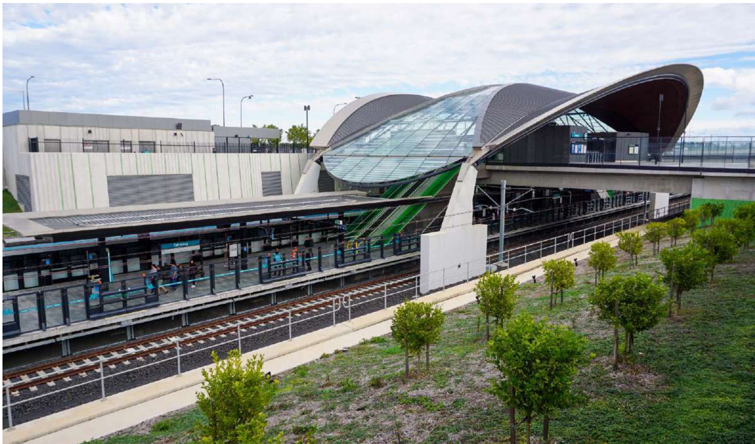
Sydney Metro: Tallawong station, the northern terminus of the current North West & Bankstown Line.
